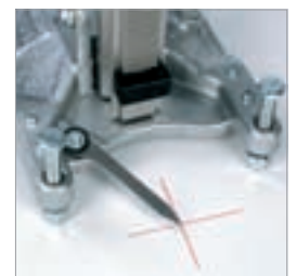
Efficient drill rig set-up using standard centralisation indicator
